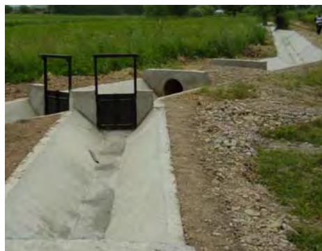
The new canal with distribution outlets in Mady village, constructed with USAID support.
